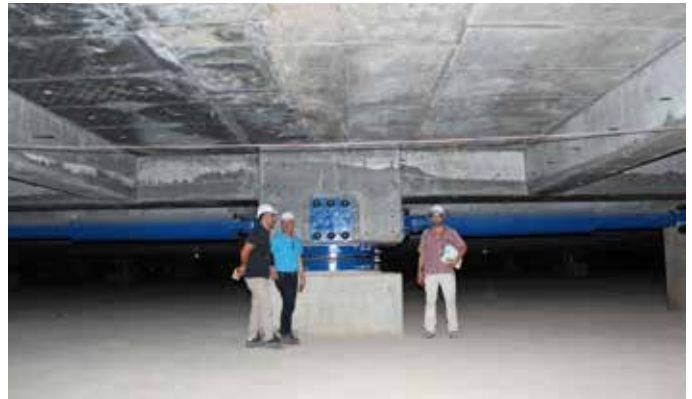
SIP Sliding Isolation Pendulum Bearing and two horizontally adaptive hydraulic dampers underneath the Mosque in Algiers. © KREBS + KIEFER Ingenieure GmbH
