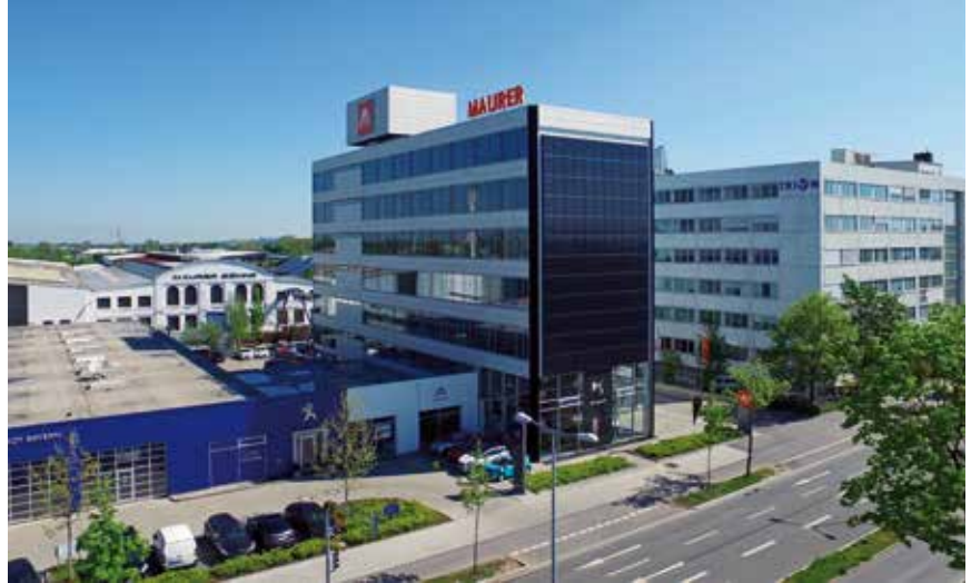
MAURER headquarters, Munich / Germany
