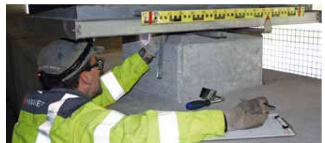
Inspection of bridge bearings
