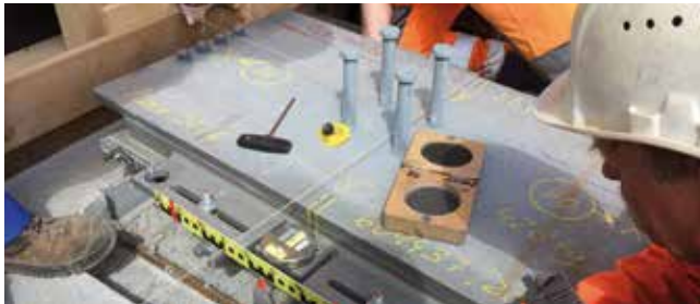
Installation Botlekbrug, Netherlands
